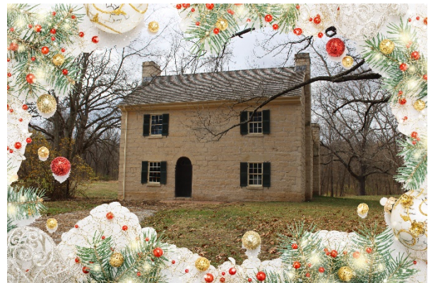
The Historic Daniel Boone Hays Home at Matson Hill Park in Defiance is opening its doors to visitors for the first time this holiday season. The new attraction will offer free candle-lit holiday tours in the park Dec. 4-5 and 11-12, 2020. The 1830s establishment was once the home of Daniel Boone's grandson and is featured on the National Register of Historic Places .
